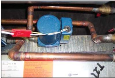
**The SureFlow heating-and-cooling system uses circulators rather than control valves for enhanced efficiency and maintenance.**
