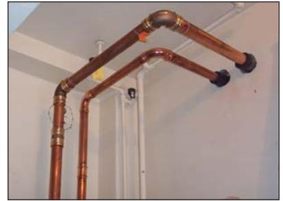
**The two-pipe system reduces the amount of pipe and fittings needed to heat and cool the classrooms and offices.**
