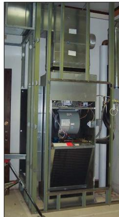
**The fan coil accommodates the circulators' relatively low pressure drop capability and results in higher than typical water flows.**
